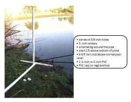
NOTE: drill a 3/8 hole in the top of each foot to allow water to enter the riser system.
